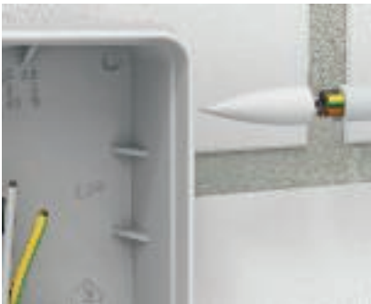
Insertion point application Place the insertion point on the end of the wire. Push the cable with the point through the pre-marked entries.
