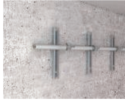
Wall mounting Cable mounting on profile rails with clamp clips.
