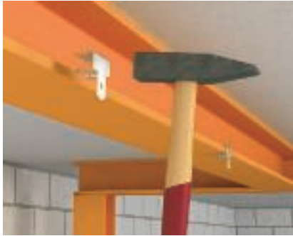
Opening of beam clamps Beam clamps are attached to the flange and they then grab it.
