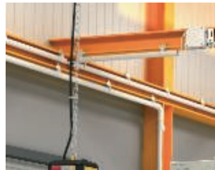
Beam clamp installation Beam clamps can be knocked onto the flange both in a horizontal and a vertical position.
