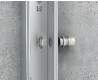
Mounting of brass cable gland The required openings are drilled in the side wall of the LKM. Then, push the cable glands through the opening and lock them tightly in the interior with a locknut.
