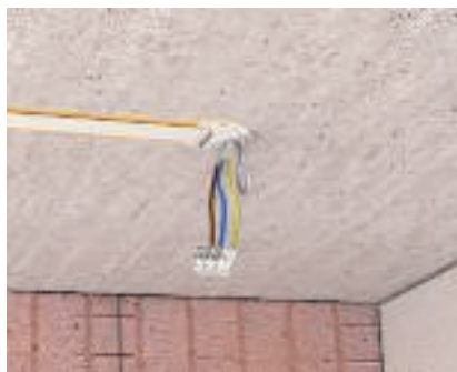
Terminal strip application For luminaire connection, wire ends can be secured with terminal clips.
