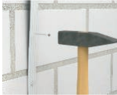
Siko nail application The Siko nail is placed in the separating retainers of the ribbon conductor.
