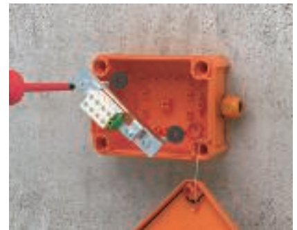
Mounting, connection unit Fasten the bolt tie with seals directly in the substrate through the clamp and base of the junction box.
