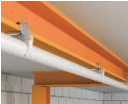
Beam clamp mounting Installation of beam clamps and installation tube parallel to flange.
