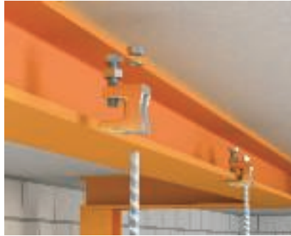
Screwing on of beam clamps Screw-in beam clamps are pushed onto the flange and the flange clamped using the bolt in the beam clamp.
