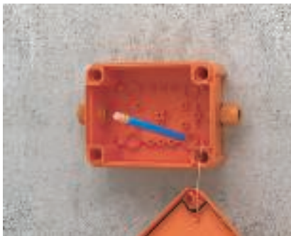
Mounting preparations Draw on the drill holes for subsequent mounting.
