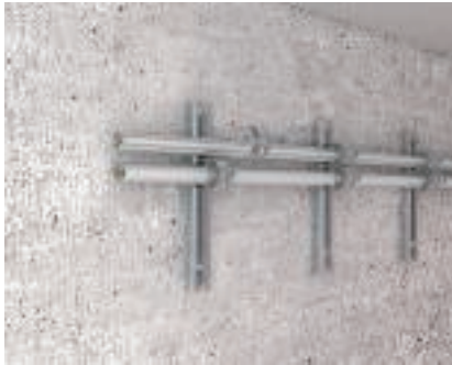
Wall mounting Cable mounting on profile rails with clamp clips.
