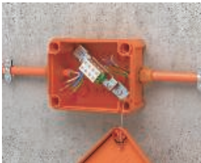
Cable insertion Strip the cable ends and insert them into the junction box through the cable gland.
