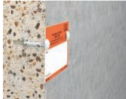
Complete installation, push-fit anchor with mushroom head 910/STP Push the push-fit anchor through the mounting section and into the drill hole.
