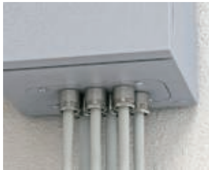
Cone cable gland application Cables can be inserted in switching systems and distributor cabinets using cone cable glands.
