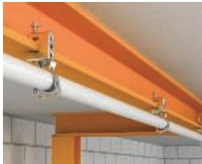
Beam clamp mounting Installation of screw-in beam clamps and installation tube parallel to flange.
