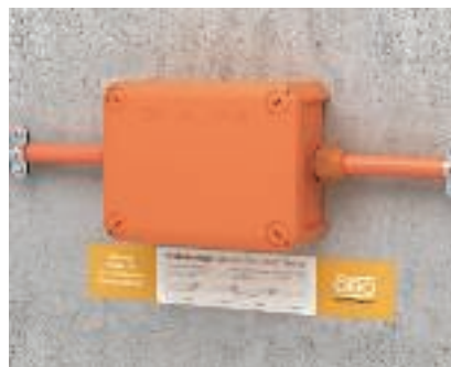
Labelling Attach the sign with the cable system data according to DIN 4102 Part 12.
