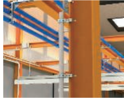
Beam clamps for pipes Use of screw-in beam clamps with directly fastened pipe seat.
