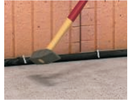
Hook nail application Knock the hook nail into the mounting substrate. Care must be taken here that the pipe is not deformed too much. For this reason, fastening cables with hook nails is critical.
