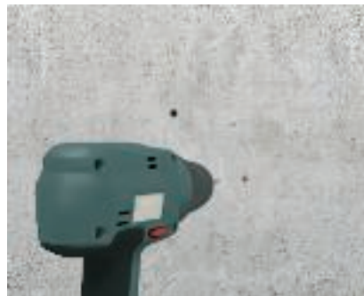
Drill fastening holes Drilling diameter: 5 mm, 60 mm deep. Clean the drill holes well.
